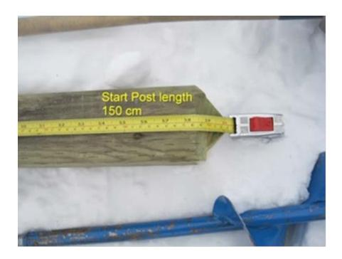
The start gate consists of two square posts, 150cm long and 9cm square. The top of the posts must be flat. The posts must be placed at the front edge of the start ramp. The area up to the front face of the posts must be level. The slope starts at the front face (course side) of the posts.
